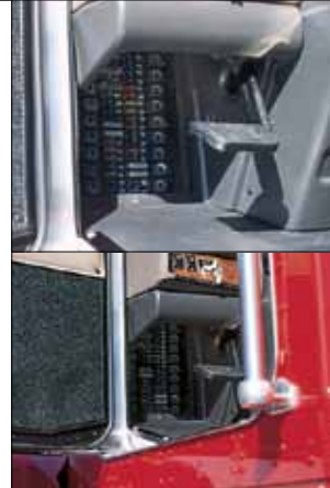
The power distribution box puts all circuit protection elements in one, central, lighted location that's close at hand.
