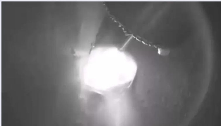
Torch misaligned to fillet joint
