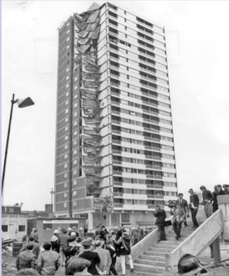
Ronan Point Collapse in North London in 1967.
