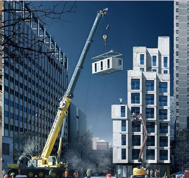
Construction of high-rise buildings using modular units on site
