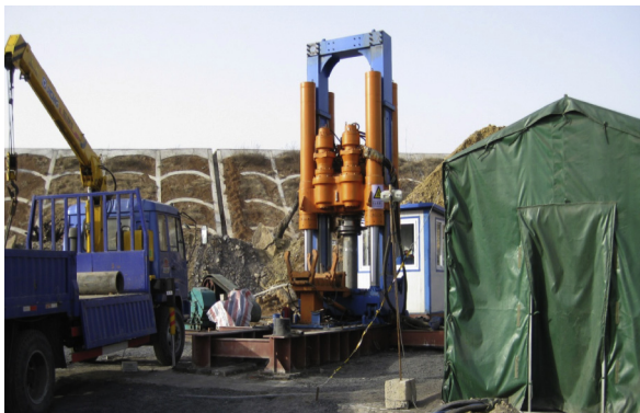
Fig. 9. Drilling site of raise boring machine.
