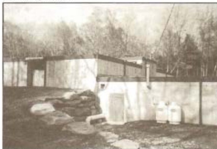
A 425,000 gpd slow sand filtration plant engineered for the Village of Woodridge, New York.
