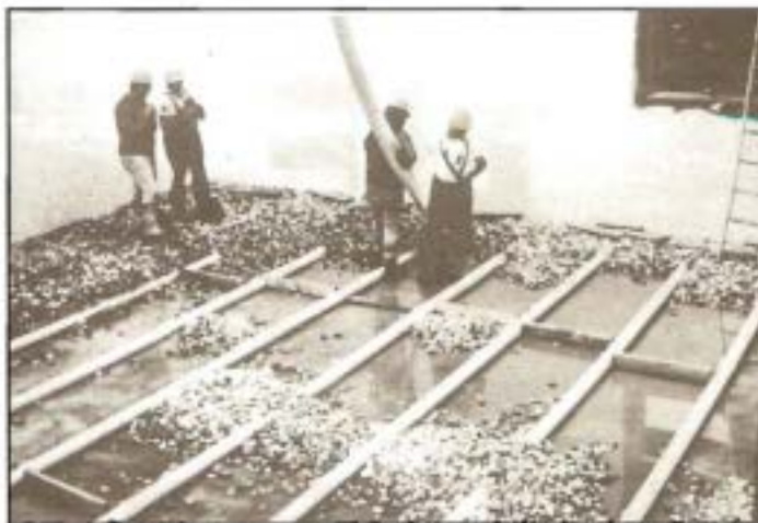
Workers install the first layer of filter media (1½ to 2½ inch diameter gravel to a depth of 8 inches) for a slow sand filtration plant in Ripley, New York.
