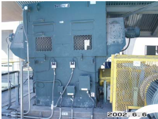
Figure 20 - 1100 hp TEBV AC VFD motor
