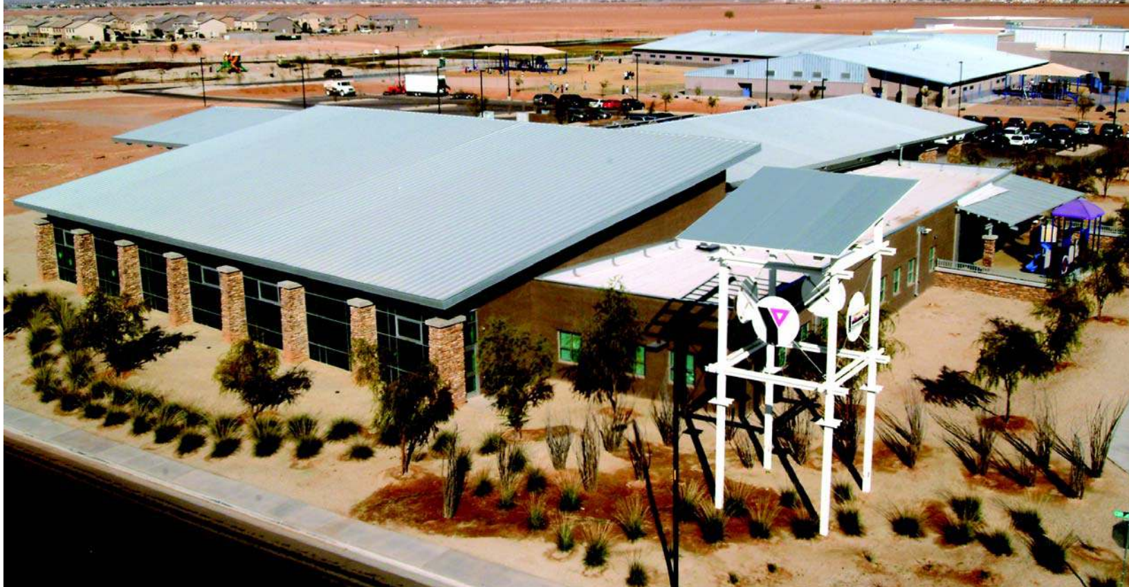
COPPER BASIN YMCA Queen Creek, Arizona
