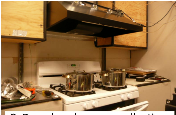
C: Deep hood; grease collection on plate, no screens.
