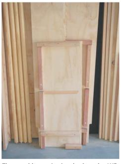
The two side panels, showing how the 1%'' x 1%'' 'ribs' have been permanently attached.
