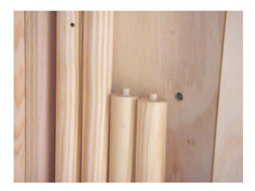
Each rod has a smaller dowel glued into the end of it – this fits into a small hole in the shelves at the top and bottom.
