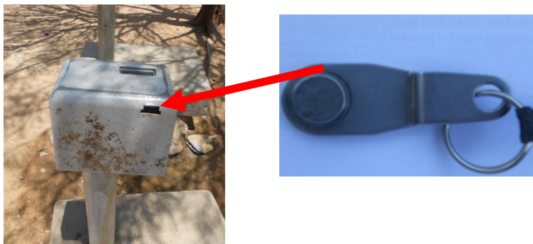
Figure 4.2: Lesira-Teq standpipe and the token used in in Karibib Usab informal settlement
