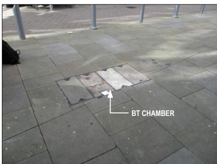
PHOTOGRAPH 1 EXISTING BT CHAMBER IN FOOTWAY ON GIBB STREET OUTSIDE BUILDING
