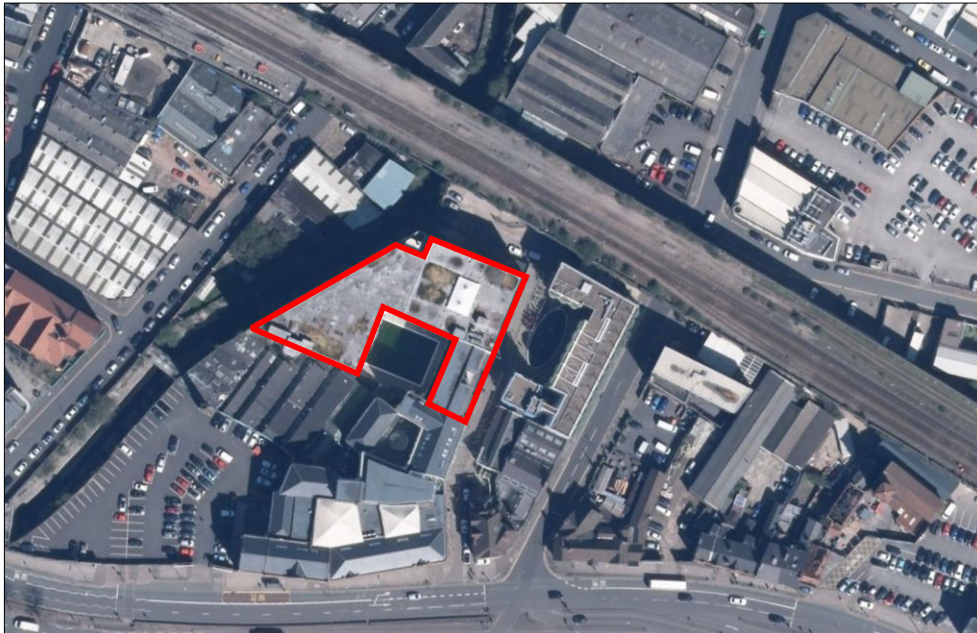
SITE AERIAL VIEW (Building highlighted in red)
