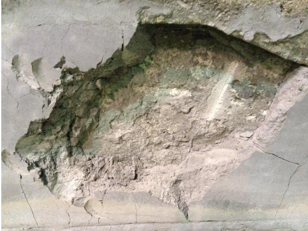
Figure 84. UNIQUE Overhead and Vertical Repair – Batch 3 bond performance
