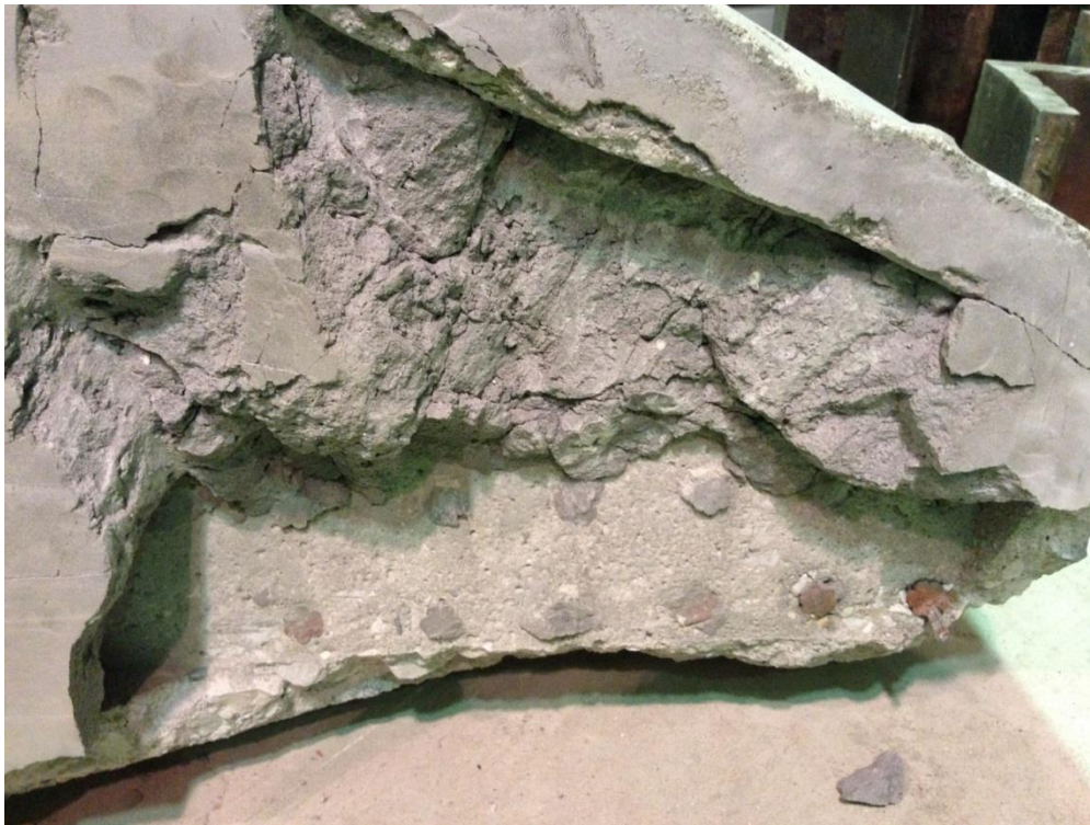
Figure 82. UNIQUE Overhead and Vertical Repair – Batch 1 bond performance
