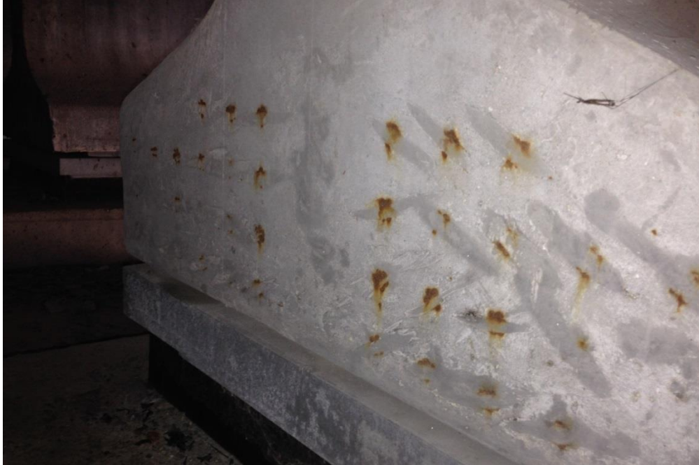
Figure 24. TEX•COTE RAINSTOPPER 140 field performance on BD13528
