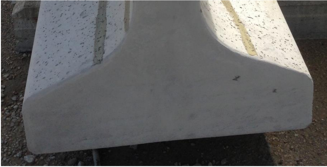
Figure 64. BD13523 before application of PAULCO TE-3008-1
