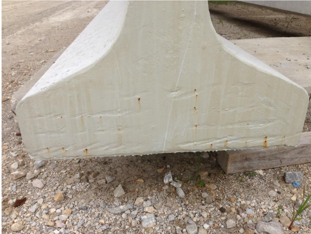
Figure 70. Beam end coated with Sikagard 62 at precast plant
