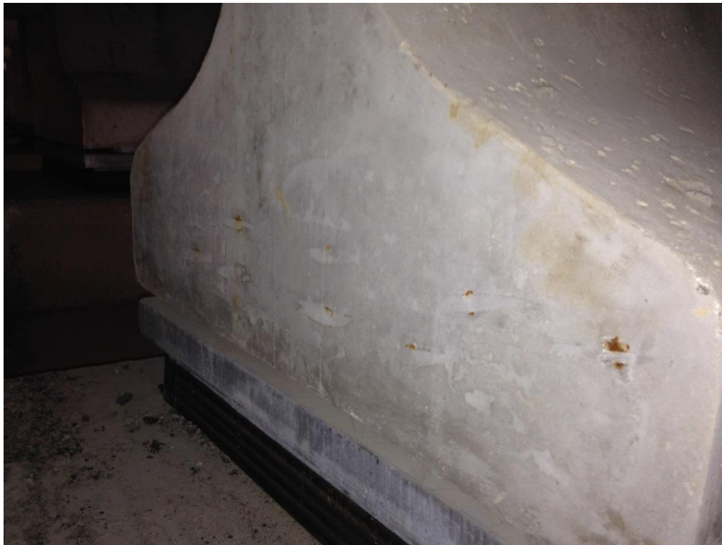
Figure 54. BASF Hydrozo 100 field performance on BD08525
