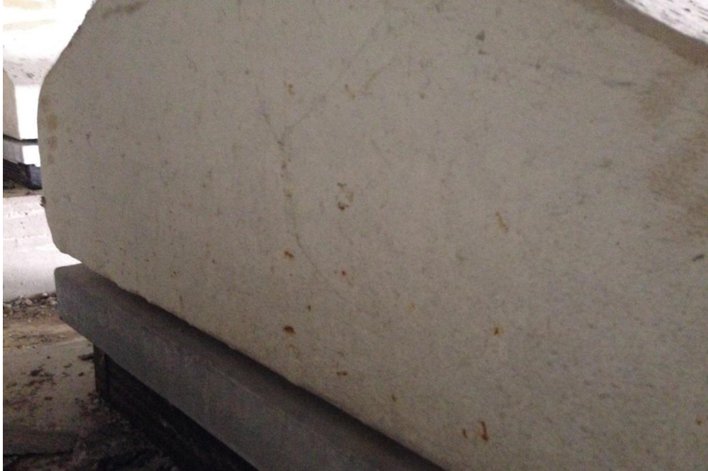
Figure 15. TEX•COTE XL 70 field condition on BD13526
