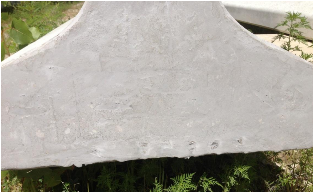
Figure 43. BD08503 before application of BASF Sonoguard
