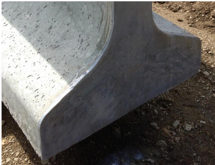
Figure 29. TEX•COTE RAINSTOPPER 140 applied to BC11526E
