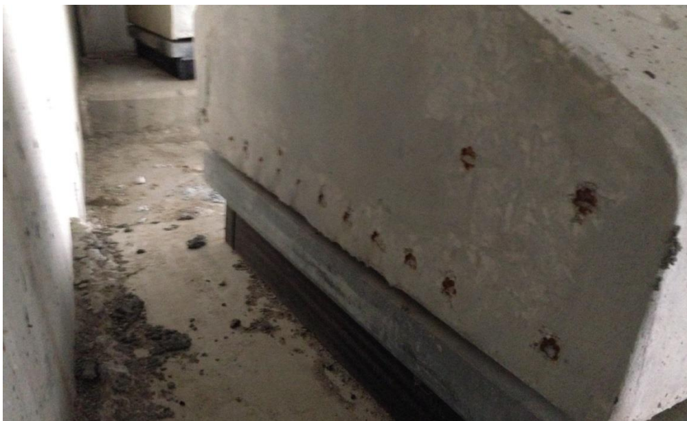
Figure 27. TEX•COTE RAINSTOPPER 140 field performance on BD08502
