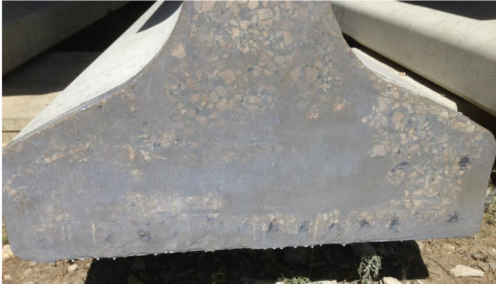
Figure 26. TEX•COTE RAINSTOPPER 140 applied to BD08502
