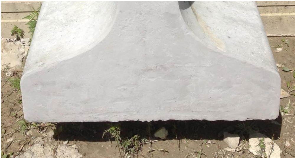
Figure 34. BD08507 prior to application of Evercrete DPS
