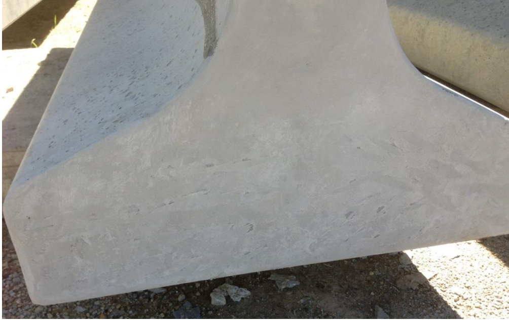
Figure 22. BD13528 prior to application of TEX•COTE RAINSTOPPER 140
