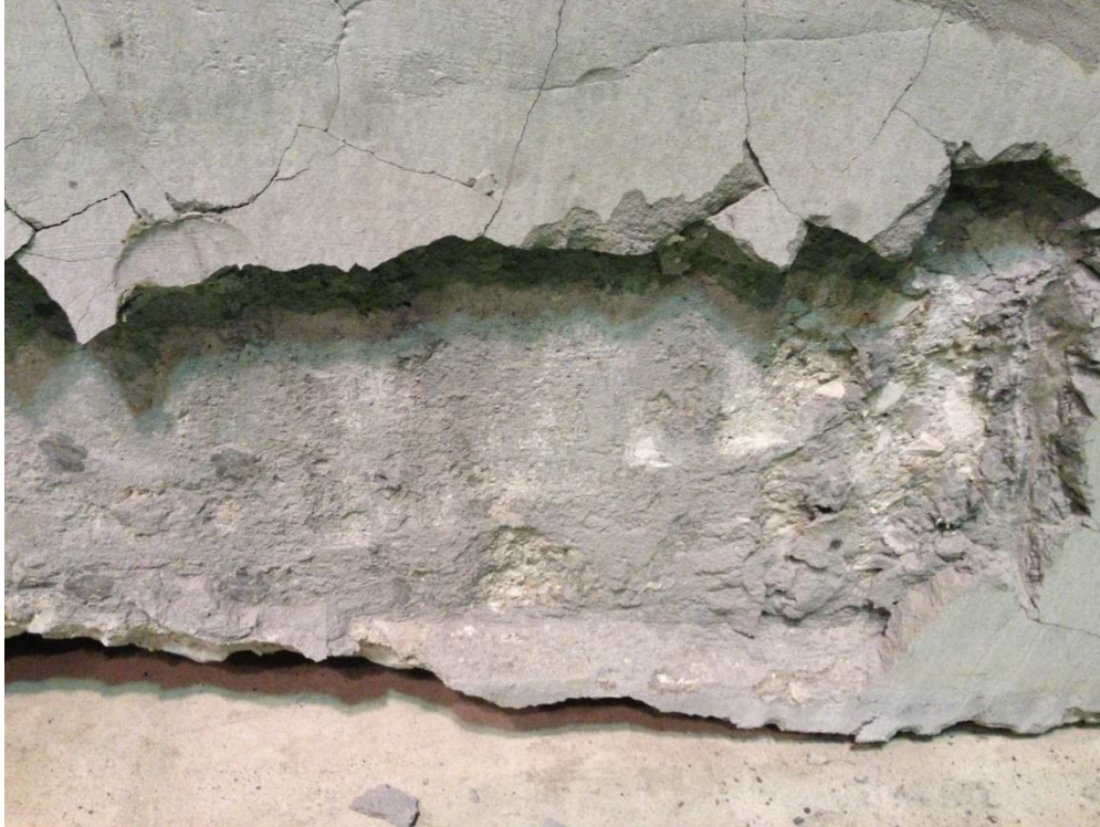
Figure 83. UNIQUE Overhead and Vertical Repair – Batch 2 bond performance
