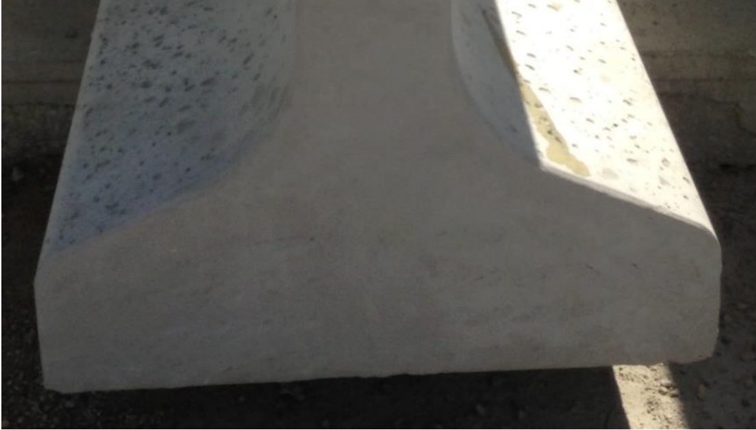
Figure 49. BD13525 before application of BASF Hydrozo 100
