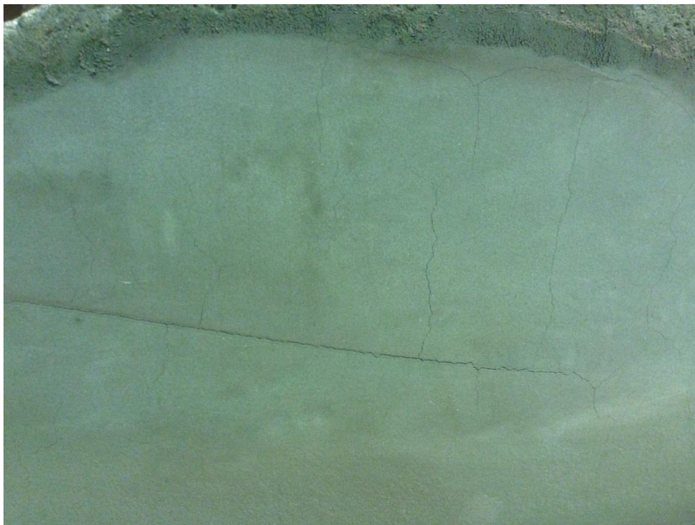
Figure 79. UNIQUE Overhead and Vertical Repair
