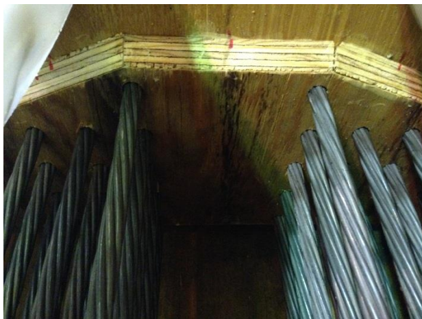
Figure 76. Single Blockout formed with \frac{3}{4} in. plywood with chamfered edges
