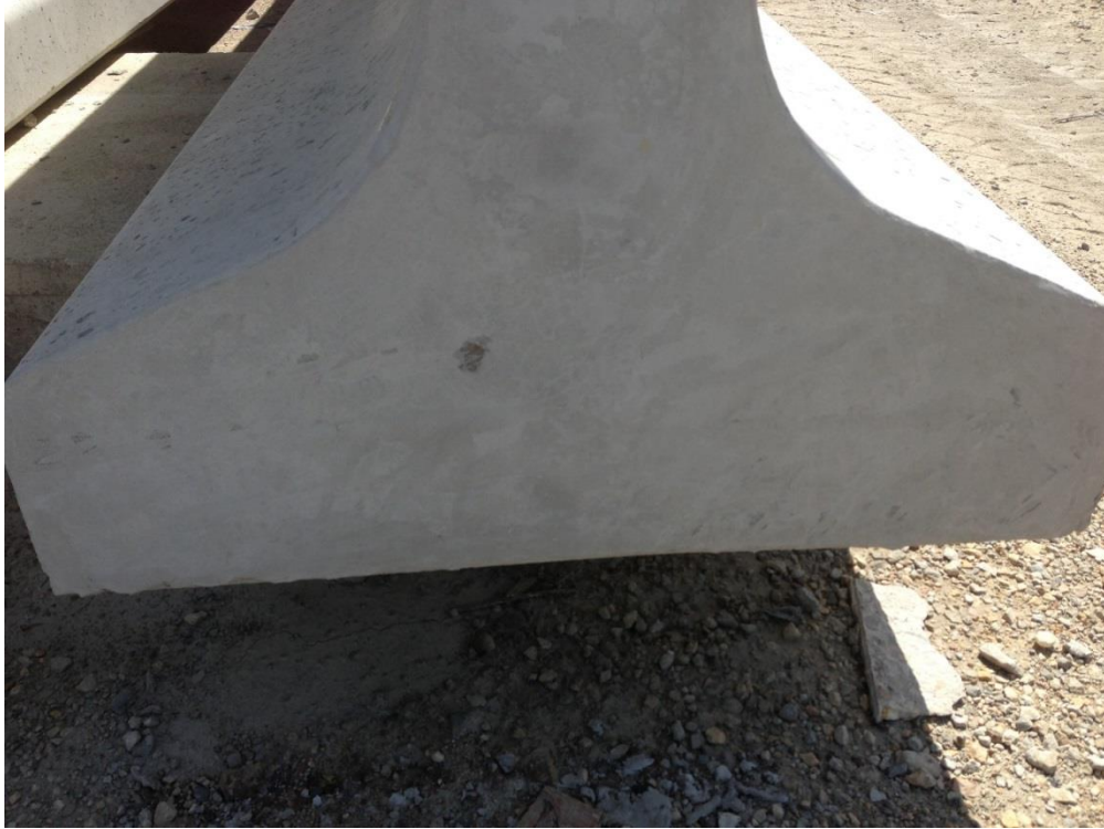
Figure 40. BD13524 before application of BASF Sonoguard
