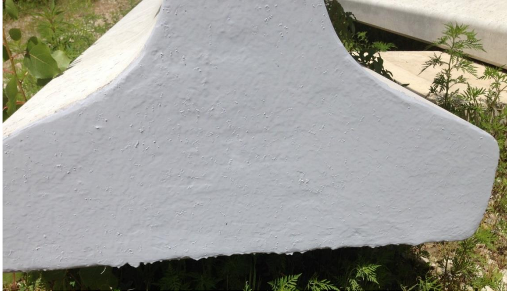
Figure 44. BASF Sonoguard applied to BD08503
