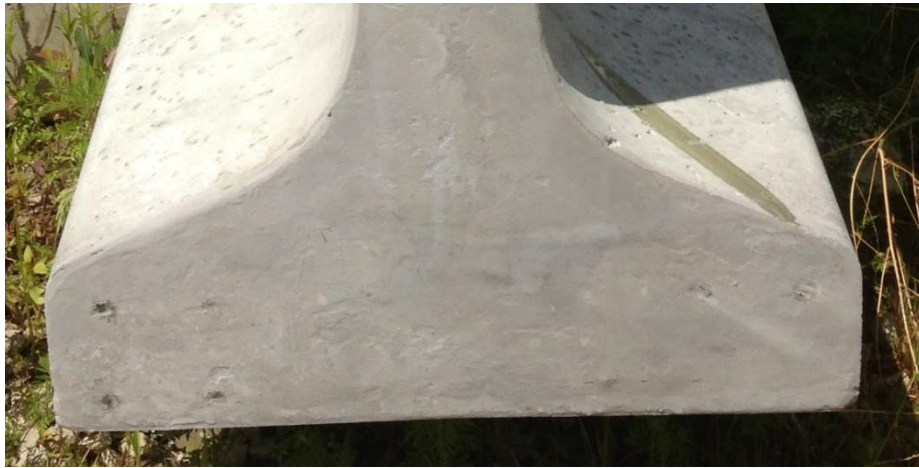
Figure 67. BD08504 before application of PAULCO TE-3008-1
