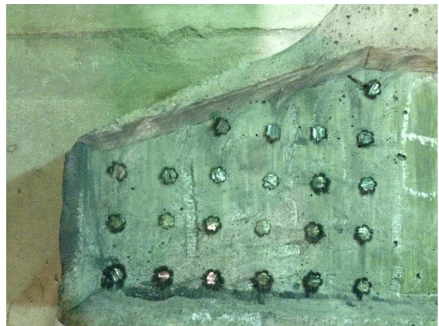
Figure 76. Single Blockout formed with \frac{3}{4} in. plywood with chamfered edges
