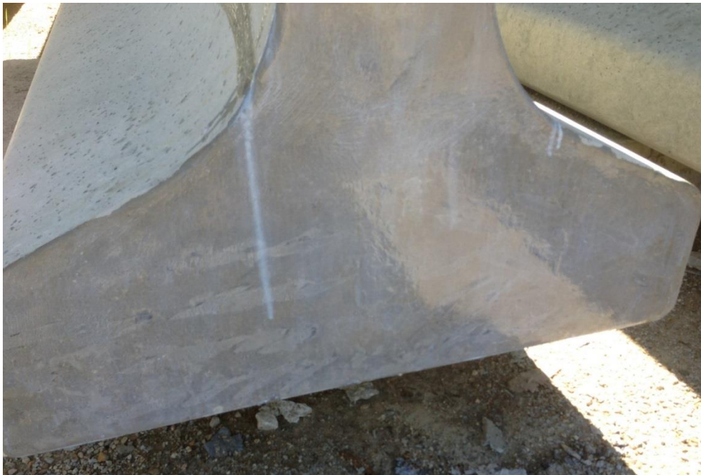
Figure 23. TEX•COTE RAINSTOPPER 140 applied to BD13528
