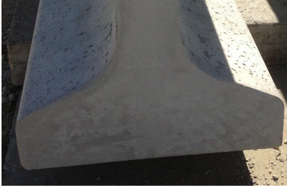
Figure 31. BD13527 prior to application of Evercrete DPS
