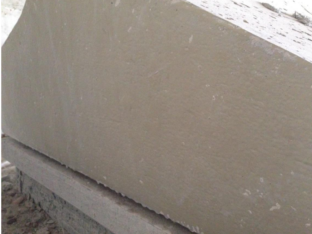
Figure 71. Good field performance of Sikagard 62 on bridge beams
