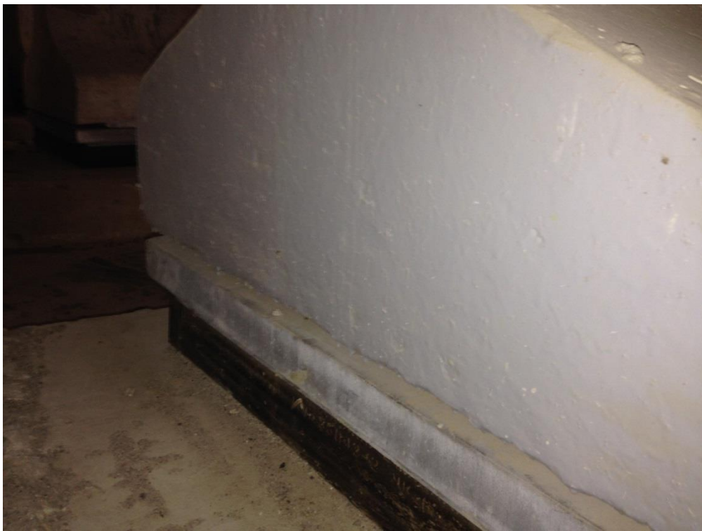
Figure 45. BASF Sonoguard field performance on BD08503
