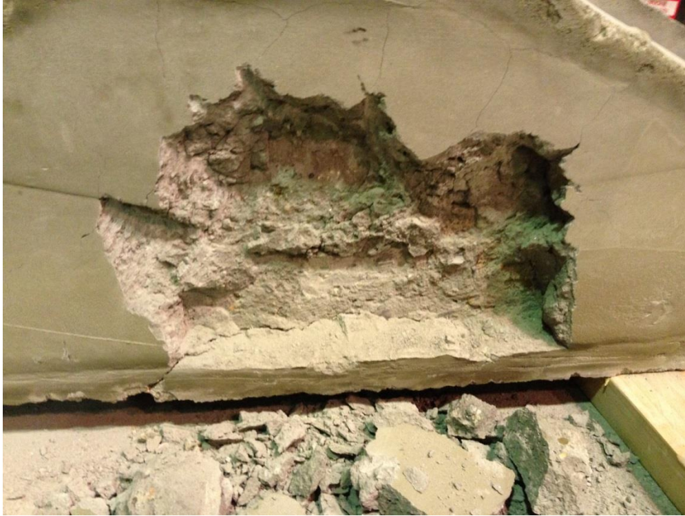
Figure 85. UNIQUE Overhead and Vertical Repair – Batch 4 bond performance
