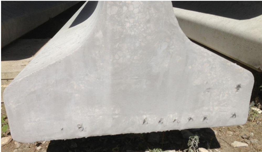
Figure 25. BD08502 prior to application of TEX•COTE RAINSTOPPER 140
