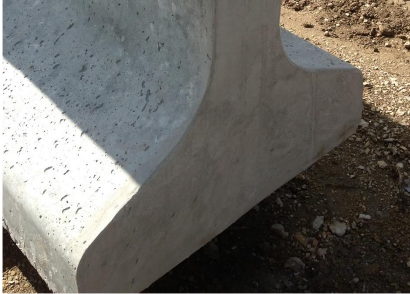
Figure 28. BC11526E prior to application of TEX•COTE RAINSTOPPER 140
