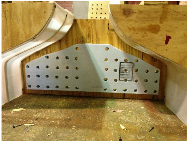
Figure 75. Single Blockout formed with 2 in. foam
