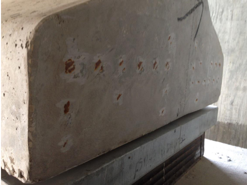
Figure 30. TEX•COTE RAINSTOPPER 140 field performance on BC11526E
