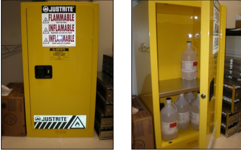
Examples of flammable storage cabinets
