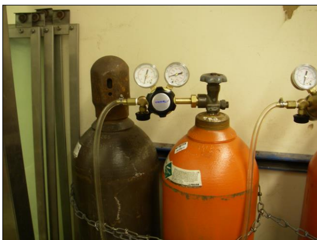
Properly attached regulator and safety cap
