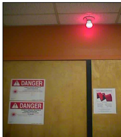
Laser warning light
