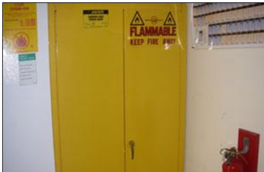
Proper storage of flammable chemicals
