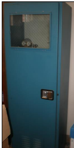
Compressed gas cylinder cabinet
