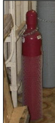
Unacceptable method of securing a gas cylinder
