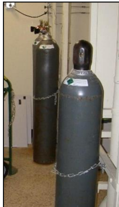
Acceptable method of securing a gas cylinder
