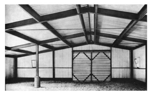
Figure 1.20 Small building made entirely of cold-formed sections. (Courtesy of Stran-Steel Corporation.) $^{1.6}$
