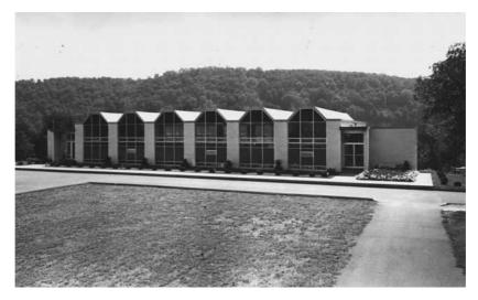
Figure 1.13 Cold-formed steel panels used in folded-plate roof. (Courtesy of H. H. Robertson Company.)
