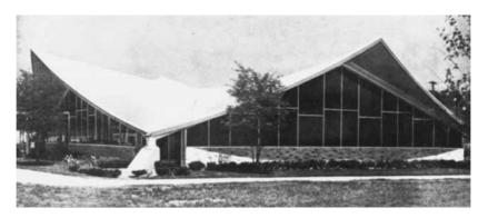
**Figure 1.14** Hyperbolic paraboloid roof of welded laminated steel deck. (Reprinted from *Architectural Record*, March 1962. Copyright by McGraw-Hill Book Co., Inc.)<sup>1.79</sup>
