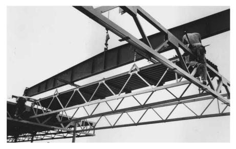
**Figure 1.17** Steel deck is designed as the top chord of prefabricated open web steel joists. (Courtesy of Inland-Ryerson Construction Products Company.)
