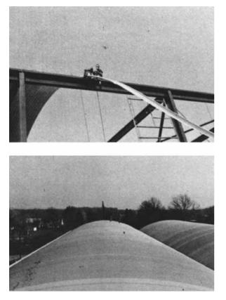
**Figure 1.16** Arched roof curved at job site. (Courtesy of Donn Products Company.)
