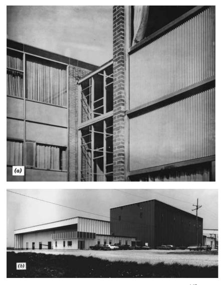
**Figure 1.18** (*a*) Exterior curtain wall panels employing corrugated steel sheets.<sup>1.87</sup> (*b*) Frameless stressed-skin construction. (Courtesy of Behlen Manufacturing Company.)
