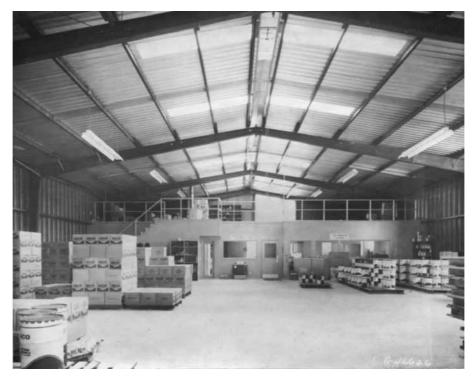
**Figure 1.21** Standardized building made of fabricated rigid frame with cold-formed sections for girts, purlins, roofs, and walls. (Courtesy of Armco Steel Corporation.)
