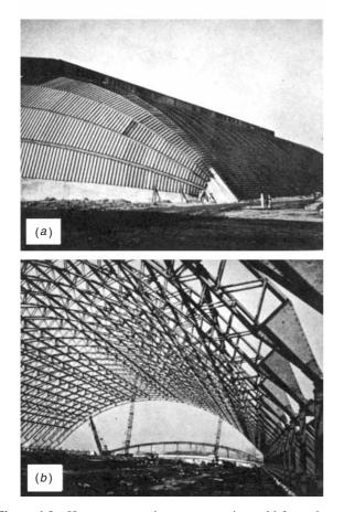
**Figure 1.9** Hangar-type arch structures using cold-formed steel sections. (Courtesy of Armco Steel Corporation.)<sup>1.6</sup>
