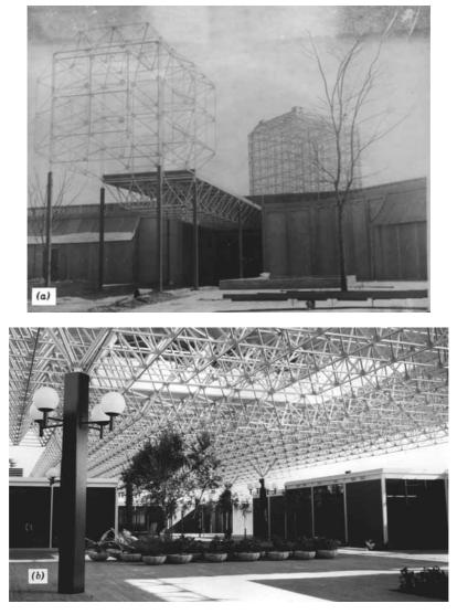
Figure 1.6 Cold-formed steel sections used in space frames. (Courtesy of Unistrut Corporation.)
