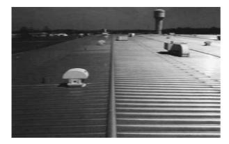
Figure 1.19 Application of standing seam roof systems. (Courtesy of Butler Manufacturing Company.)
