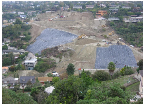
Remediation work from the 2005 Bluebird Canyon Landslide.
