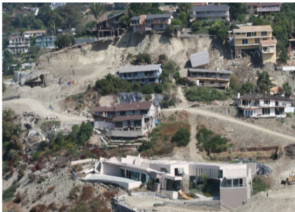
Aftermath of a massive landslide in Bluebird Canyon in 2005
