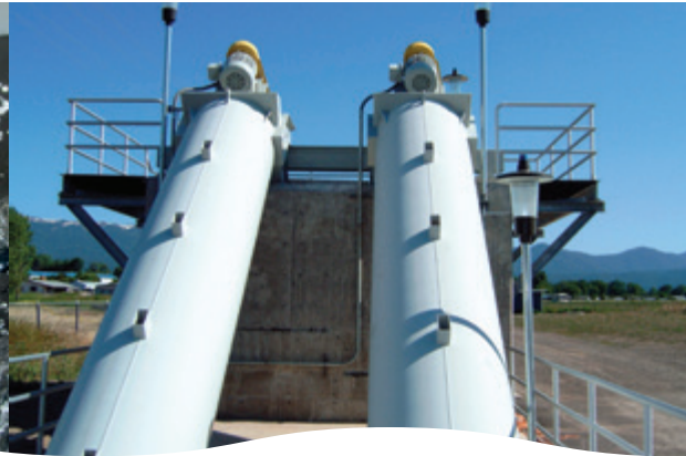
Type "S" Screw Pump Tube Vents
