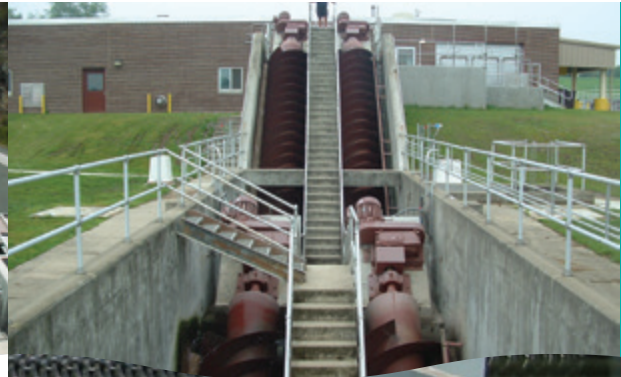
Open Screw Pump – Dual Stage Design
