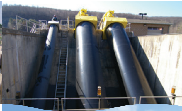
Type "C" Enclosed Screw Pump
