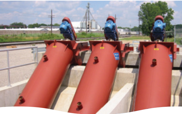
Type "S" Enclosed Screw Pump
