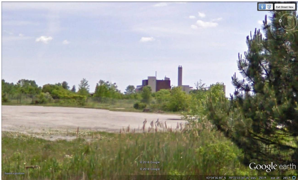
Figure C8: G.E. Booth (Lakeview) Wastewater Treatment Plant
