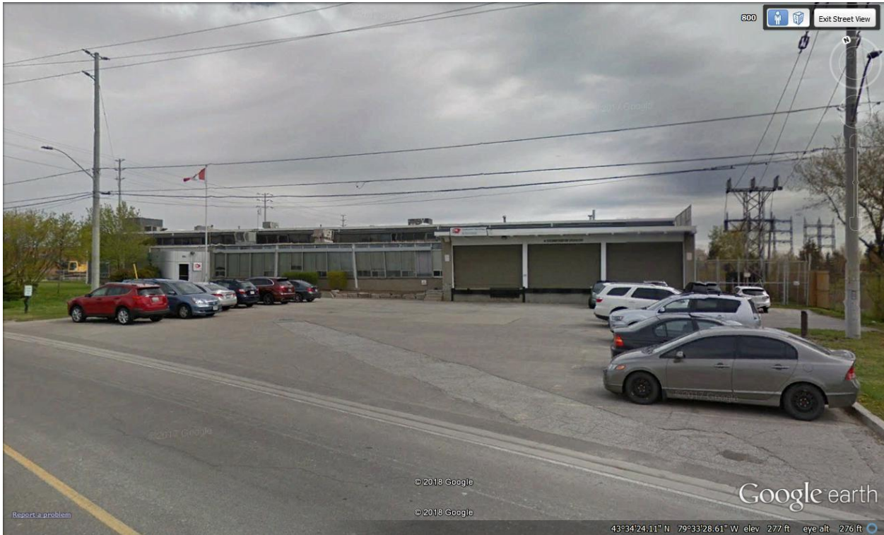
Figure C6: C/S Construction Specialties Company, 895 Lakefront Promenade
