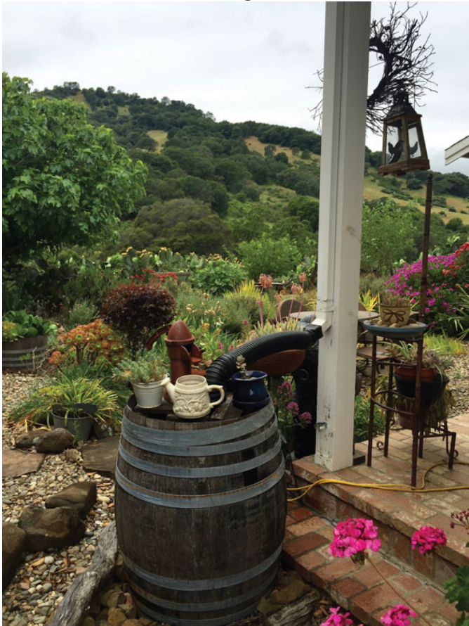
A wine barrel collects roof runoff.
