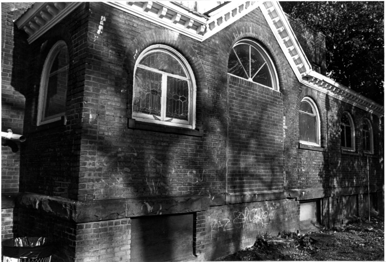
New Utrecht Reformed Dutch Church Parish House, Front facade detail
