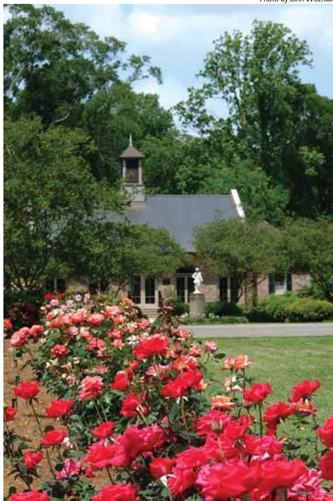
The All-American Rose Garden is in front of the Orangerie at the Burden Center. This building was designed by A. Hayes Town, a famous Baton Rouge architect, now deceased.
