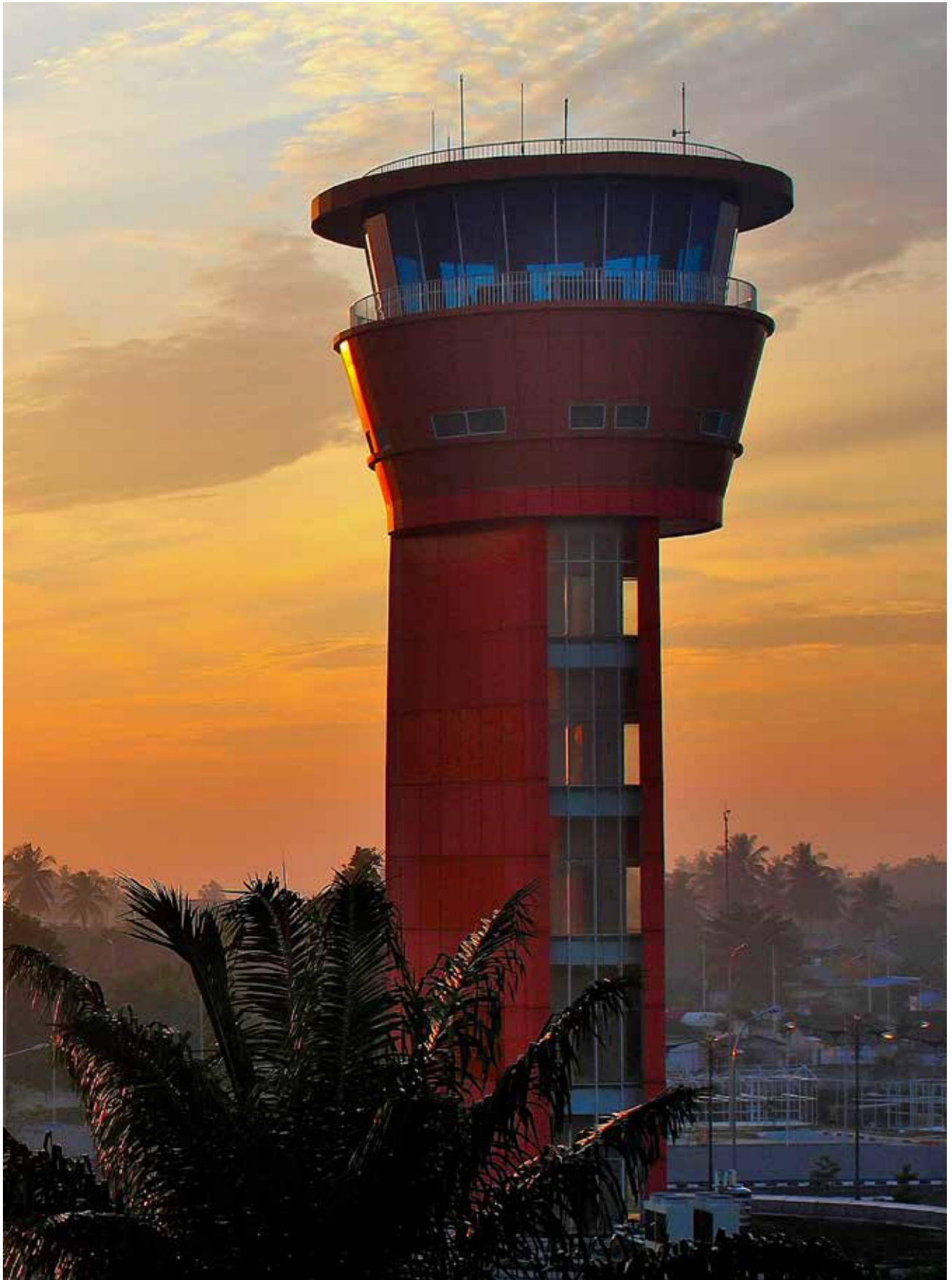
Menara ATC di Kantor Cabang Pekanbaru, Riau. ATC Tower in Pekanbaru Branch Office, Riau.
