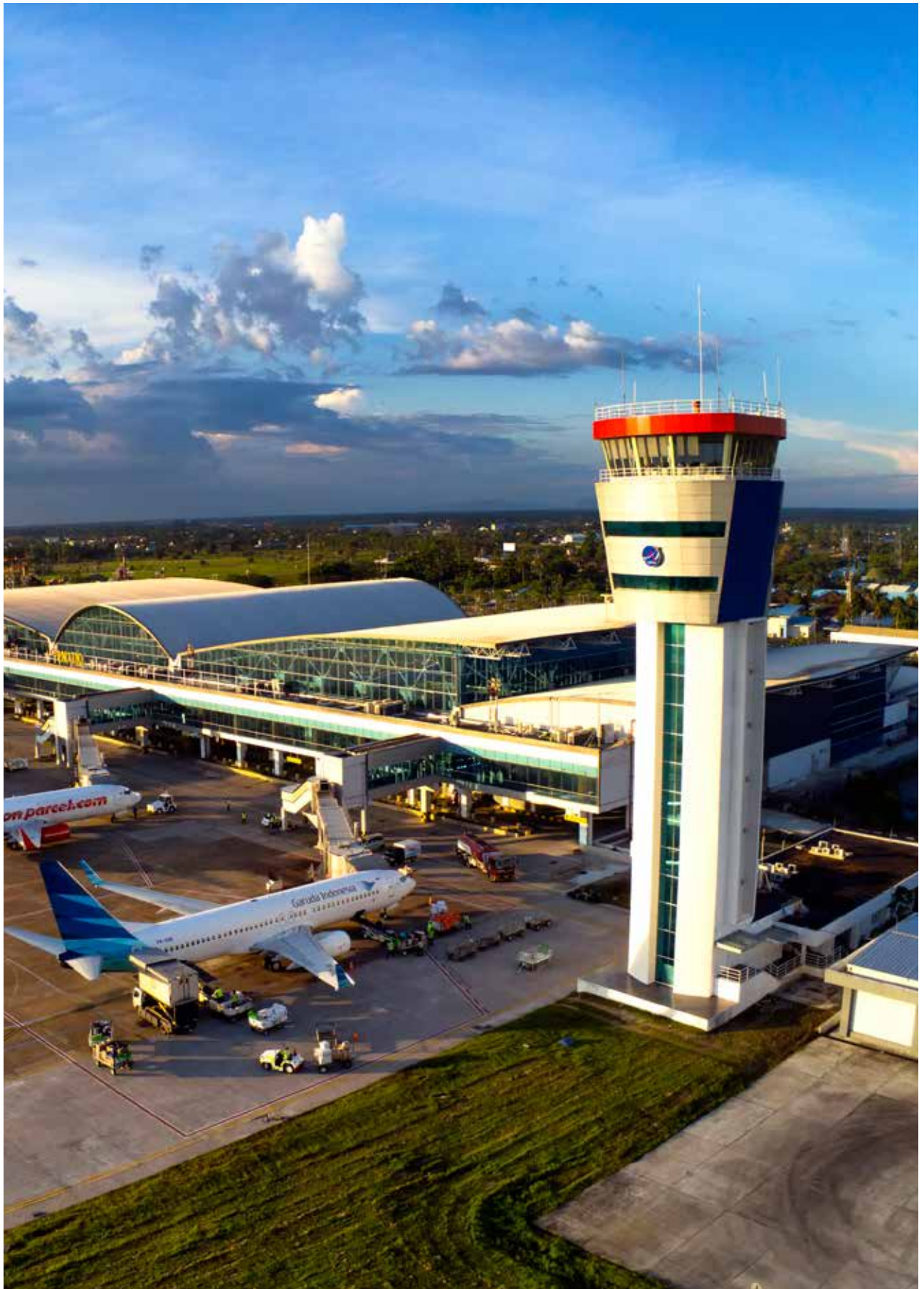
Menara ATC di Kantor Cabang Pontianak, Kalimantan Barat. ATC Tower in Pontianak Branch Office, West Kalimantan.
