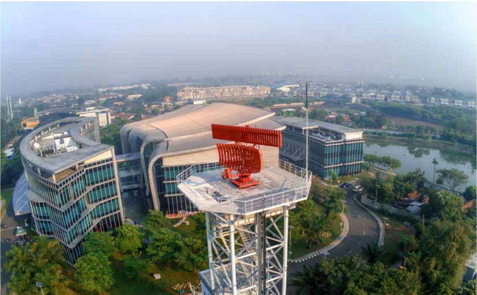
Foto udara Kantor Pusat AirNav Indonesia. Aerial view of AirNav Indonesia Head Office.
