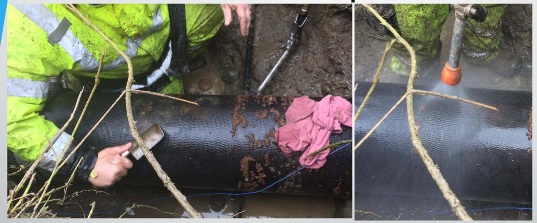
This step is very important because if you get any debris in between the pipe and the band you will not get the proper seal you need.
