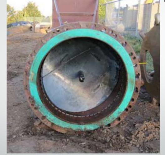
The coupon is the portion of the main that is cut out and will be on the pilot bit. This must be retrieved.
