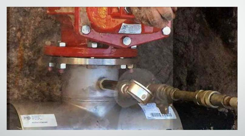
Before tapping hook up a gauge and air test the sleeve to at least the main line pressure.
