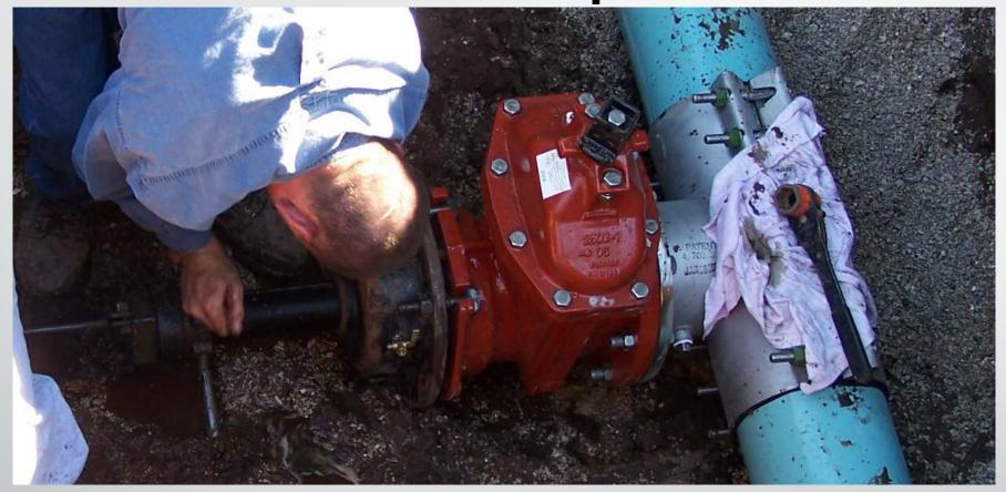
Don't be in a rush! You only go half a turn on the star for every three rotations of the bit. Continue until you hit the stop nut. Then back the bit all the way out while it is still rotating.
