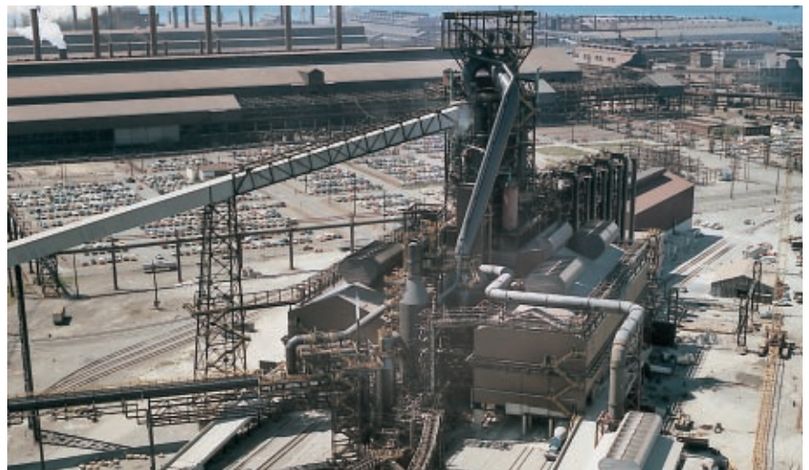
Bethlehem Steel Corporation at Sparrows Point, MD, USA
