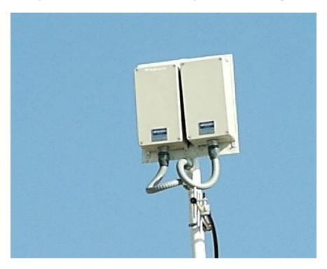
NOTE: Receivers and repeaters should not be mounted on metal fixtures
