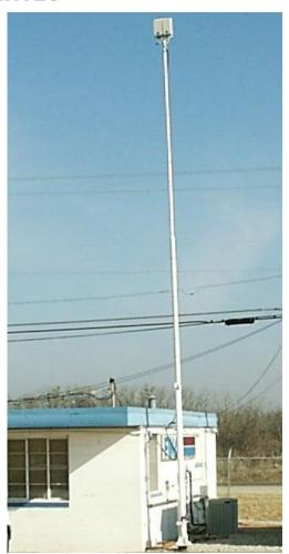
Installation with a mast which can be lowered for maintenance
