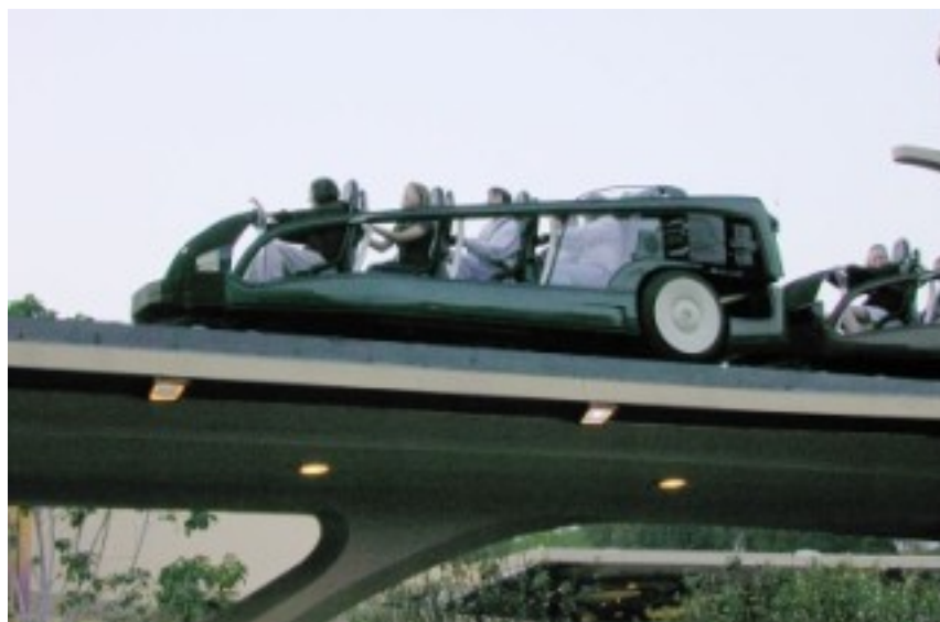
Disneyland's Rocket Rods on the elevated structure they permanently damaged.
