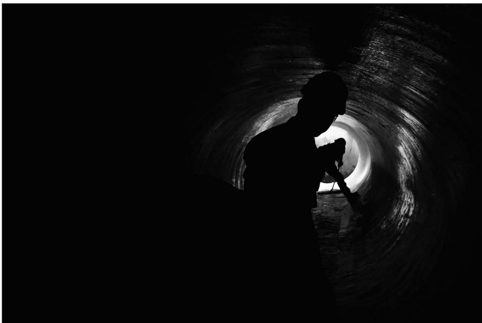
Maj. Michael Knauf looks on as Dusty Pickens sweeps water in raw water pipes near the Engine Test Facility J-3 test cell at Arnold Air Force Base during a Sept. 23 inspection of pipes recently lined with a fiber-reinforced polymer. (U.S. Air Force photo by Bradley Hicks)
