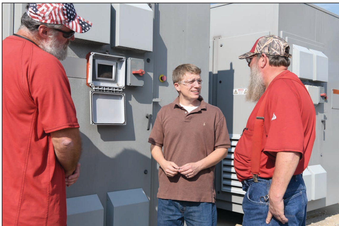
Electricians Lon Britt, left, and Robert Campbell, right, along with electrical engineer Adam Webb look at a rectifier, like one that was responsible for an un-commanded "runaway" condition, outside the AEDC Aerodynamic and Propulsion Test Unit at Arnold Air Force base. Webb improved the logic used in the Programmable Logic Controllers on the units to handle un-commanded "runaways," which allowed him to identify the part at fault. (U.S. Air Force photo by Jill Pickett) (This image has been altered by obscuring items for security reasons.)
