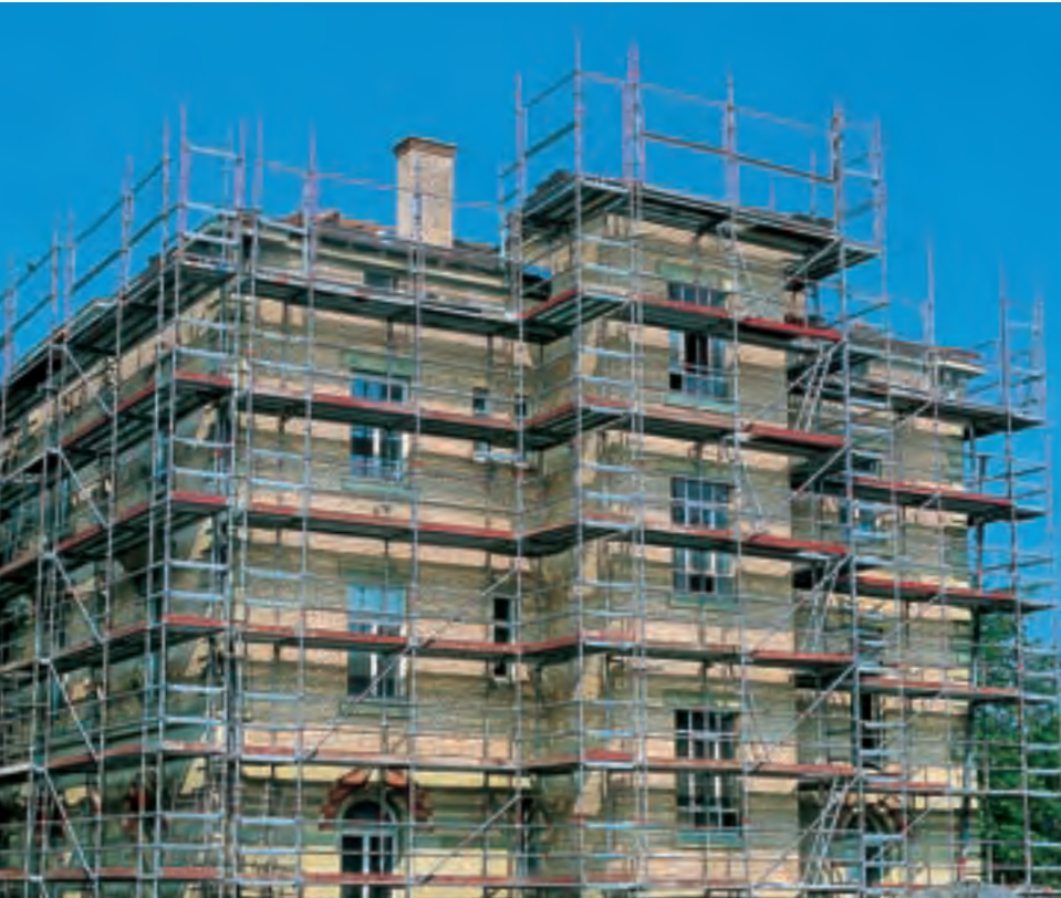
Facade scaffolding for heavily structured facades
