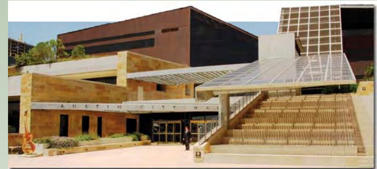
Austin's angular city hall earned a gold LEED rating for its innovative design and energy-saving features. Most of the building materials were chosen for their high degree of recycled content. On the plaza, a large solar panel generates 9 kilowatts a day and shades seating during outdoor events. Photo by Douglas Falls, TCEQ
