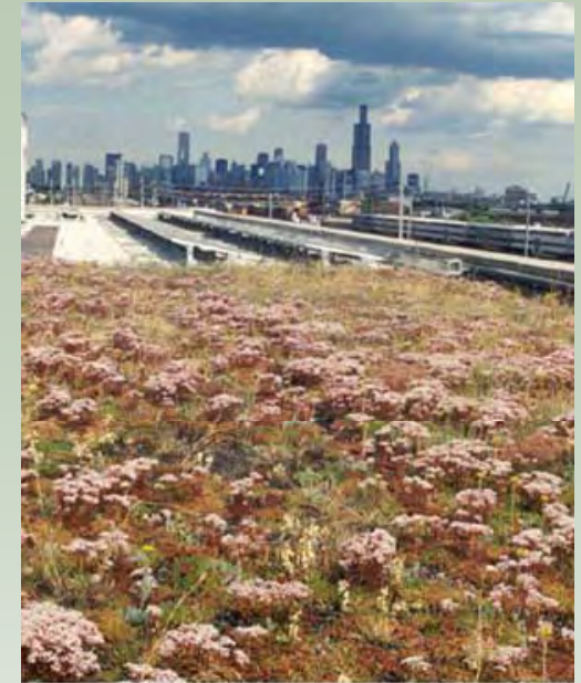
Green Roof at Chicago Center for Green Technology
