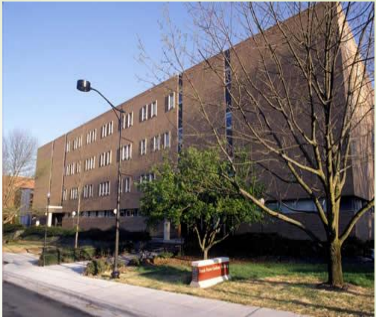
Frank Porter Graham Building Built 1970 Contains 14 classrooms and three academic departments 67,403 GSF
