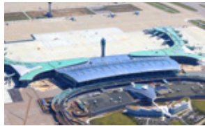
3 rd PHASE CONSTRUCTION (2009~2017) Terminal 2, Access road, and Railway
