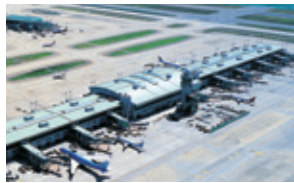
2 nd PHASE CONSTRUCTION (2002~2008) Concourse, Runway 3
