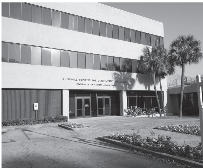
Regional Center for Continuing Education Building
