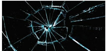
Cracked glass more than 1/2" in diameter or spidered cracks
