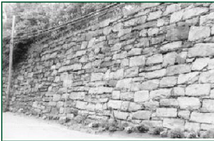
. Semi Gravity Retaining Wall
