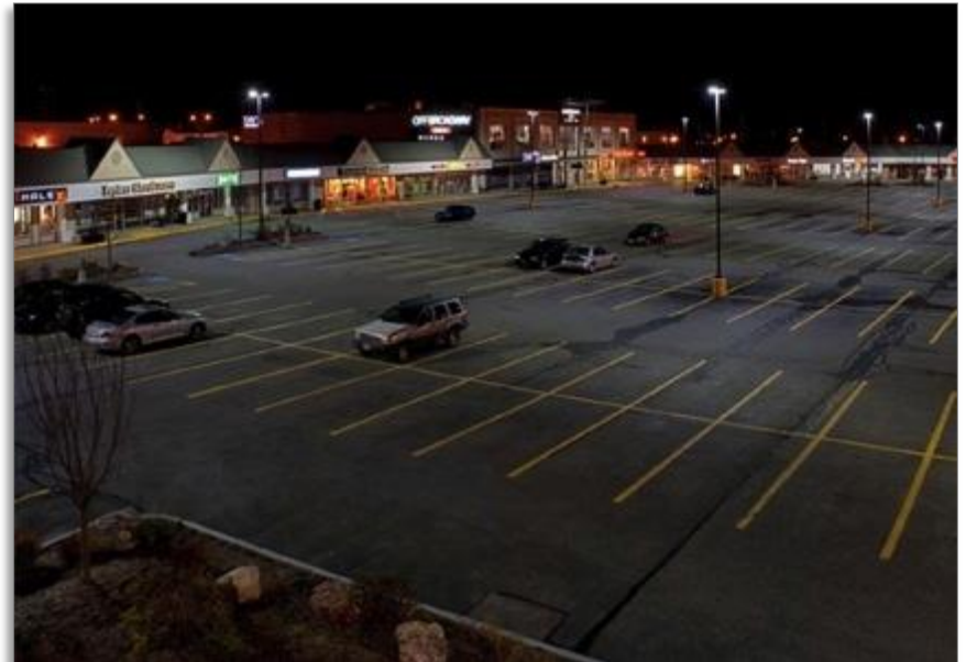
Retrofit with LED, High Power
