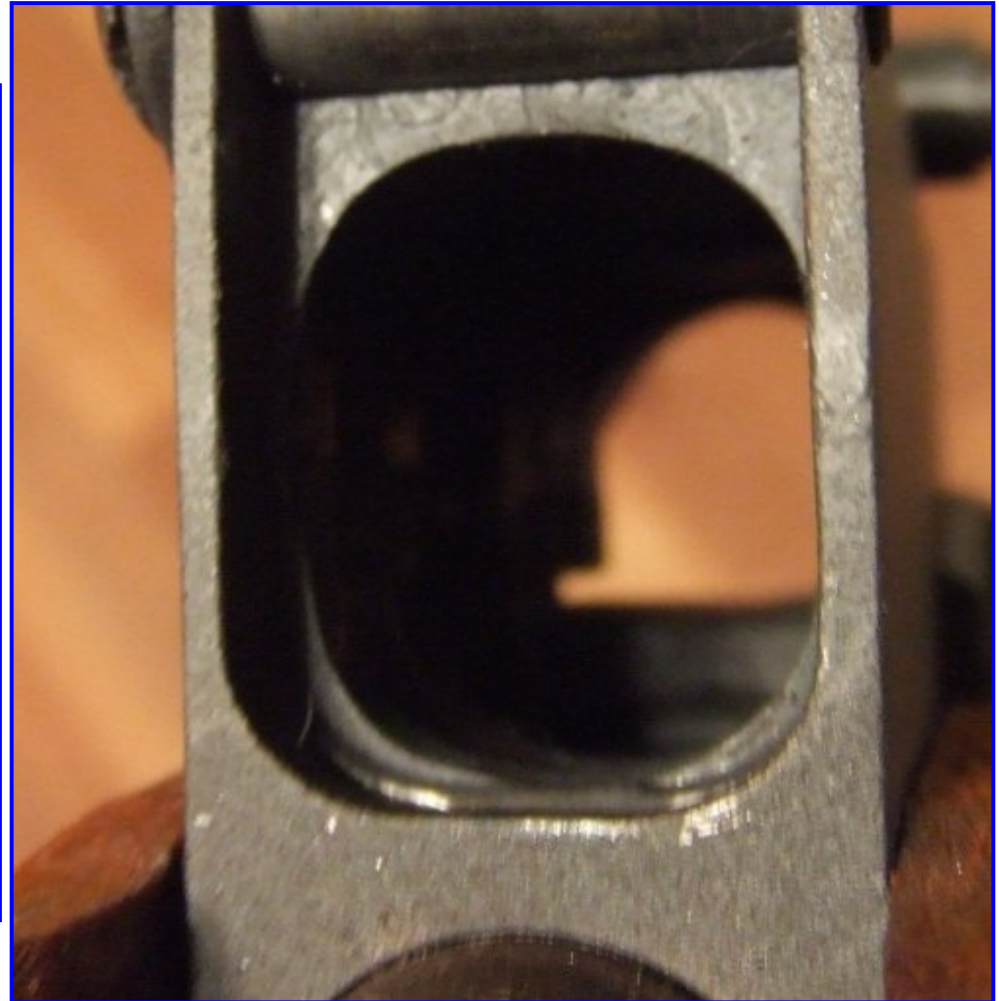
Right: AK-47 gas piston hole through upper portion of front trunion.
