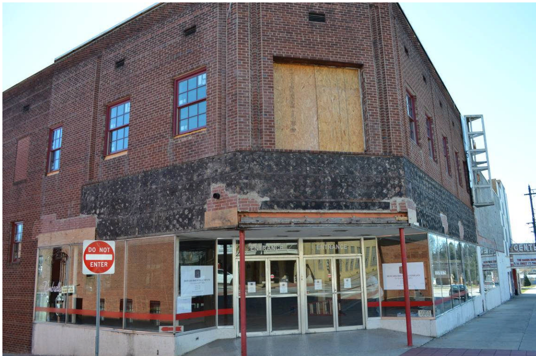
O. P. Lutz Furniture Company and Lutz Hosiery Mill, 1001 West Avenue
