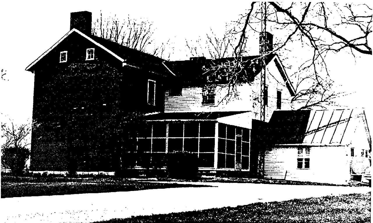
Illustration 3 Deputy Commander's quarters (Building 29), Blue Grass Facility, view from the west (top) and from southeast (bottom). This two-story brick house located on the west side of the Blue Grass site was built c. 1811 and is largely intact. The outline of the original porch can be seen in the upper photograph. (Source: Field inventory photograph, 1983, William A. Brenner, Building Technology, Inc.)
