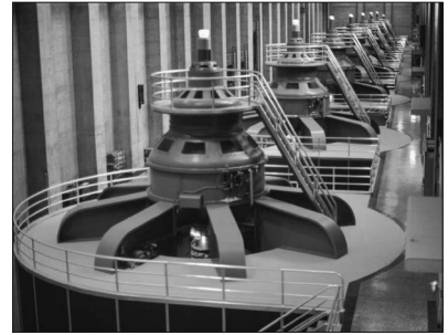
This power plant at the Hoover Dam in Nevada uses the energy from falling water to generate electrical energy.
