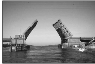
When the drawbridge is open, cars can't travel across it. In the same way, when a circuit is open, electrons can't flow through it.
