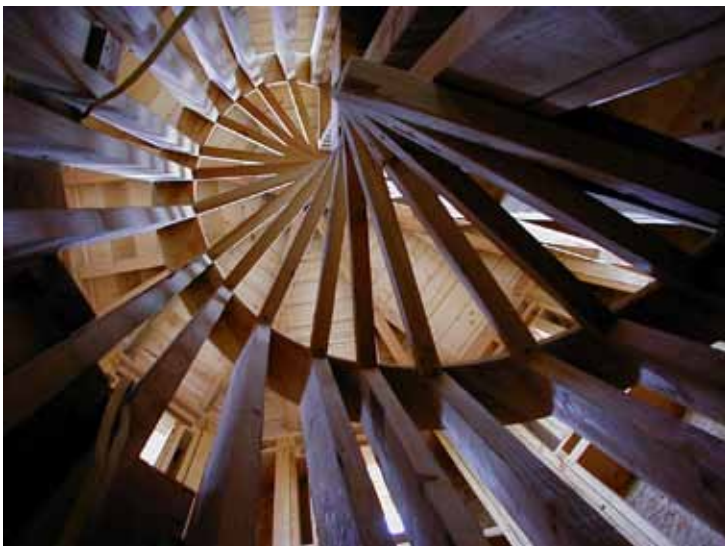
Interior construction of stair tower
