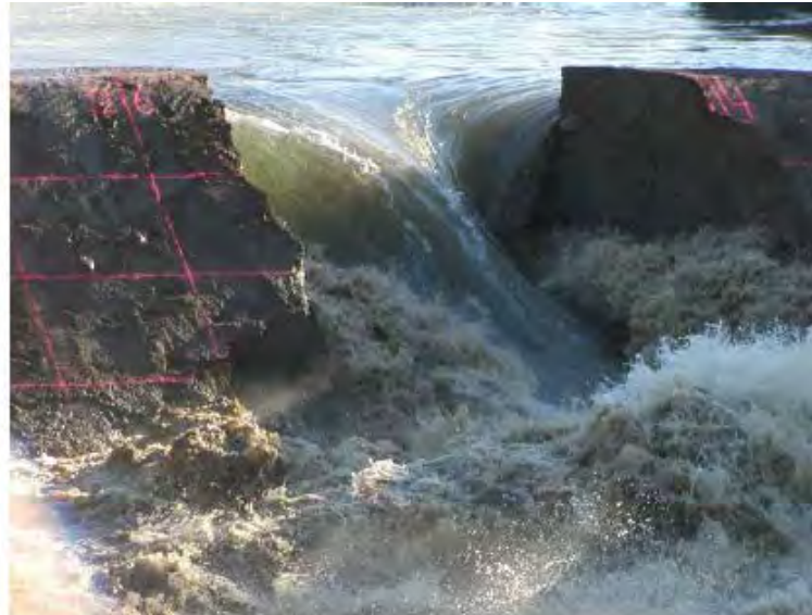
d. Flow vortices and undercutting along the toe of each eroding breach face
