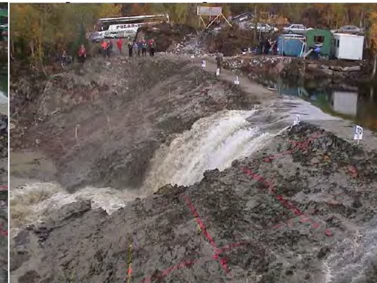
c. Progressive erosion back of headcut from toe (12:32)
