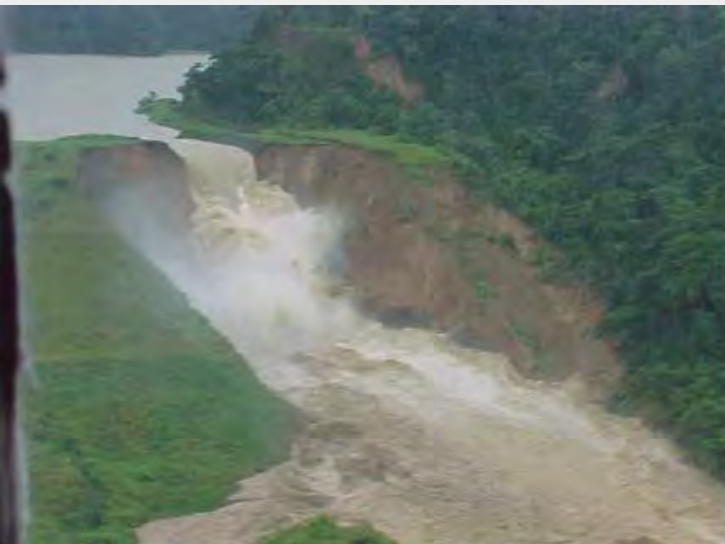
a. Headcut erosion back through dam after failure of the spillway (El Guapo Dam, Venezuela)
