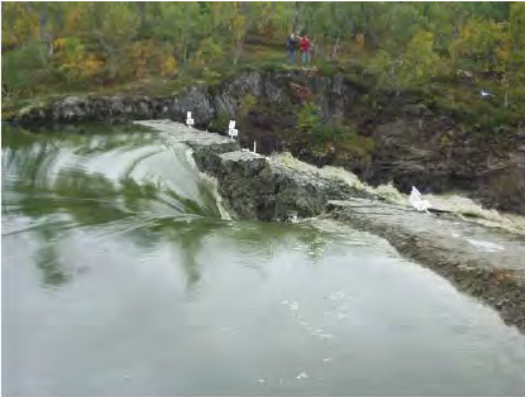
c. Flow converging to point shortly after erosion cuts through upstream crest
