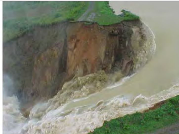
b. Vortices undercutting the breach sides just after failure of the spillway crest (El Guapo Dam, Venezuela)
