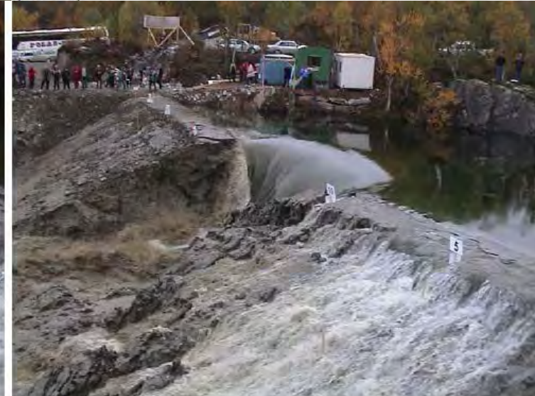
f. Failure of upstream crest / slope (13:03)
