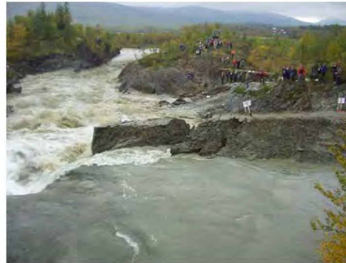
b. Tension cracks develop into block failure. Pressure of flow sliding and rotating blocks
