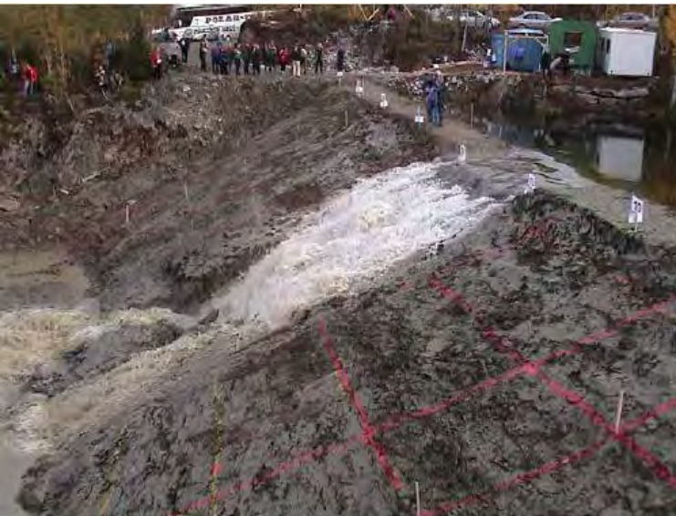
a. Initial stages of headcut formation (11:55) – erosion at weak point near toe of slope
