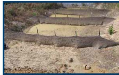
Temporary Rock Sediment Dam, Type B 1634.02 89
