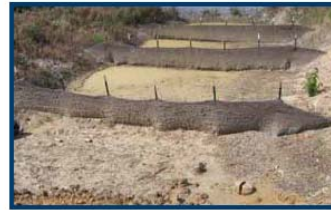
Temporary Rock Sediment Dam, Type B 1634.02
