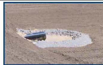
Rock Pipe Inlet Sediment Trap, Type A 1635.01
