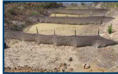
Temporary Rock Sediment Dam, Type B
