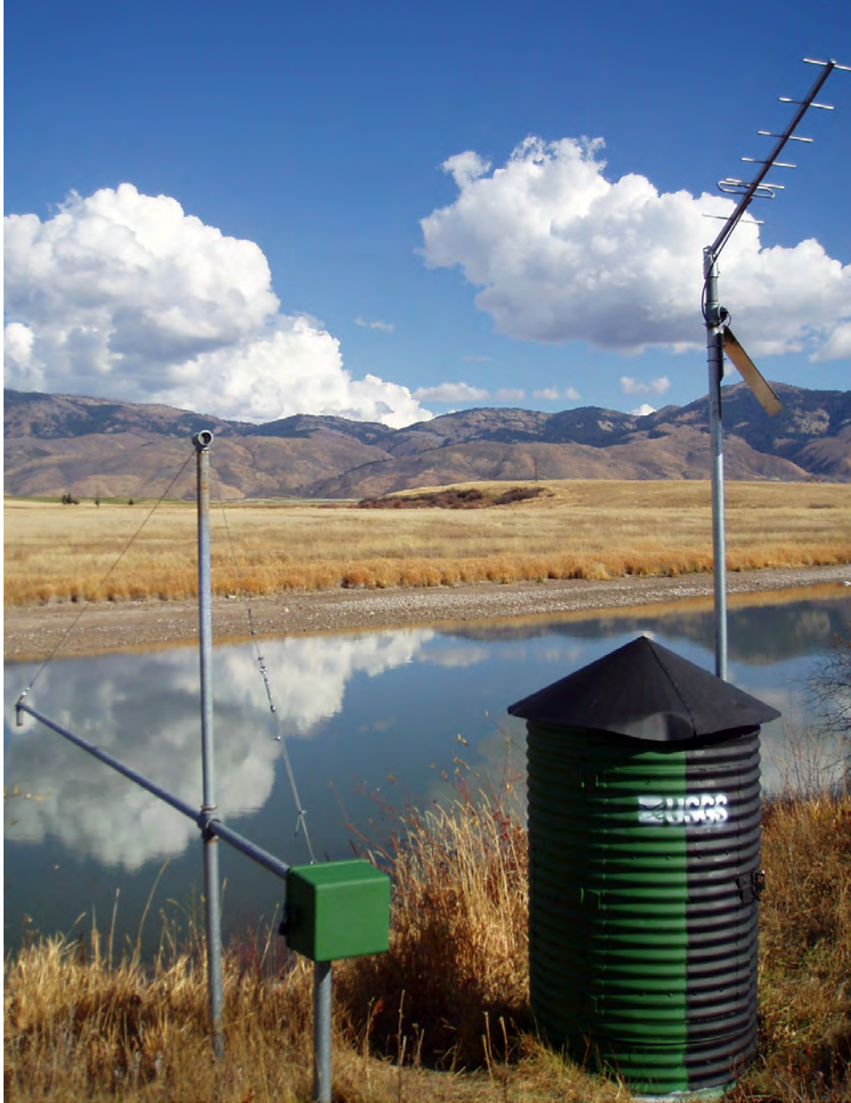
Figure 20. Cantilevered wire-weight gage located to the left of a stilling well.
