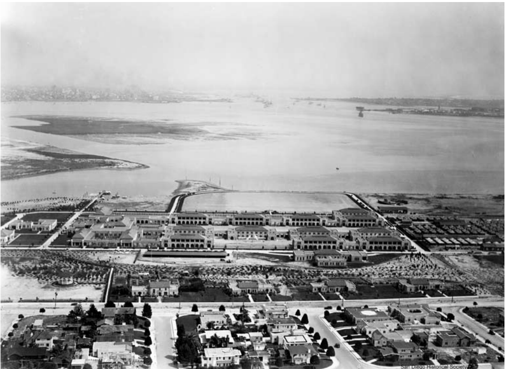
Aerial photograph of the Naval Training Station, ca. 1930. ©SDHS OP #12423-1133.
