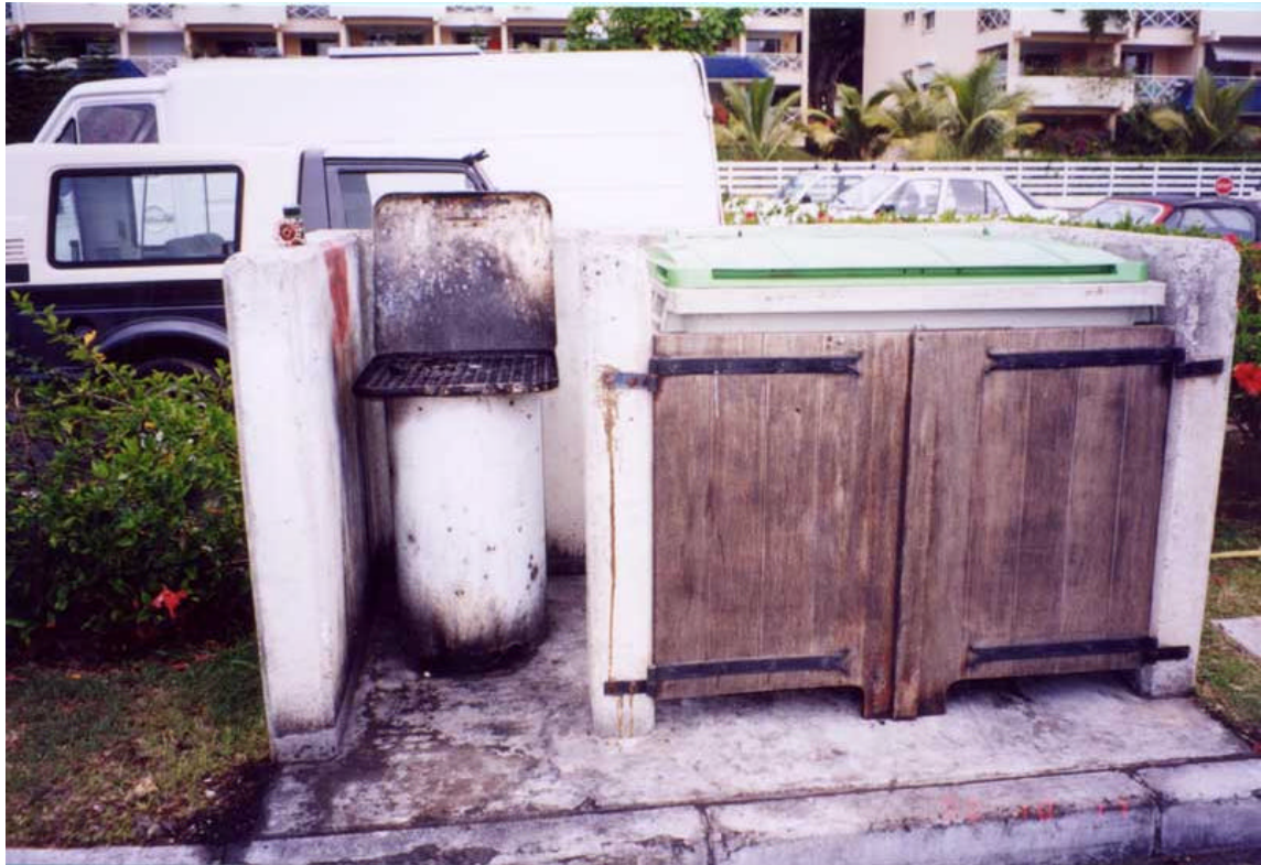
Plate 7: Garbage and Waste Oil Collection Facilities at a Small Boat Harbour in Noumea
