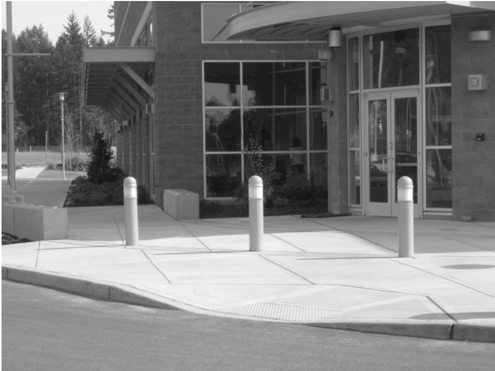
Figure 2-6 Bollards control motor vehicle traffic and block entry to protected areas
