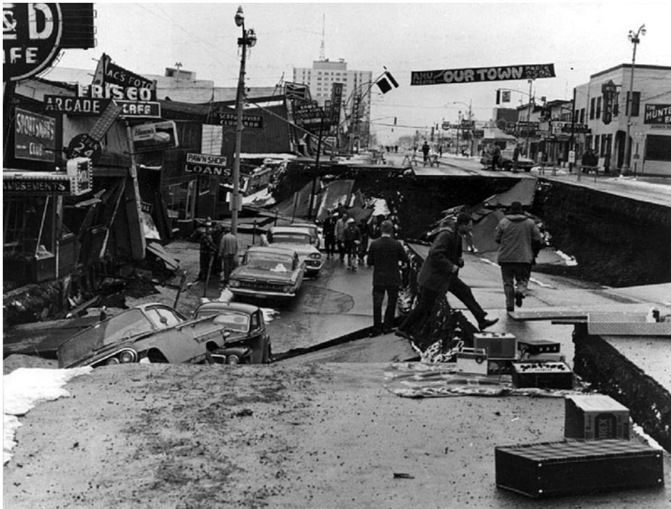
Figure 4-1 Roadway and buildings damaged in an earthquake
