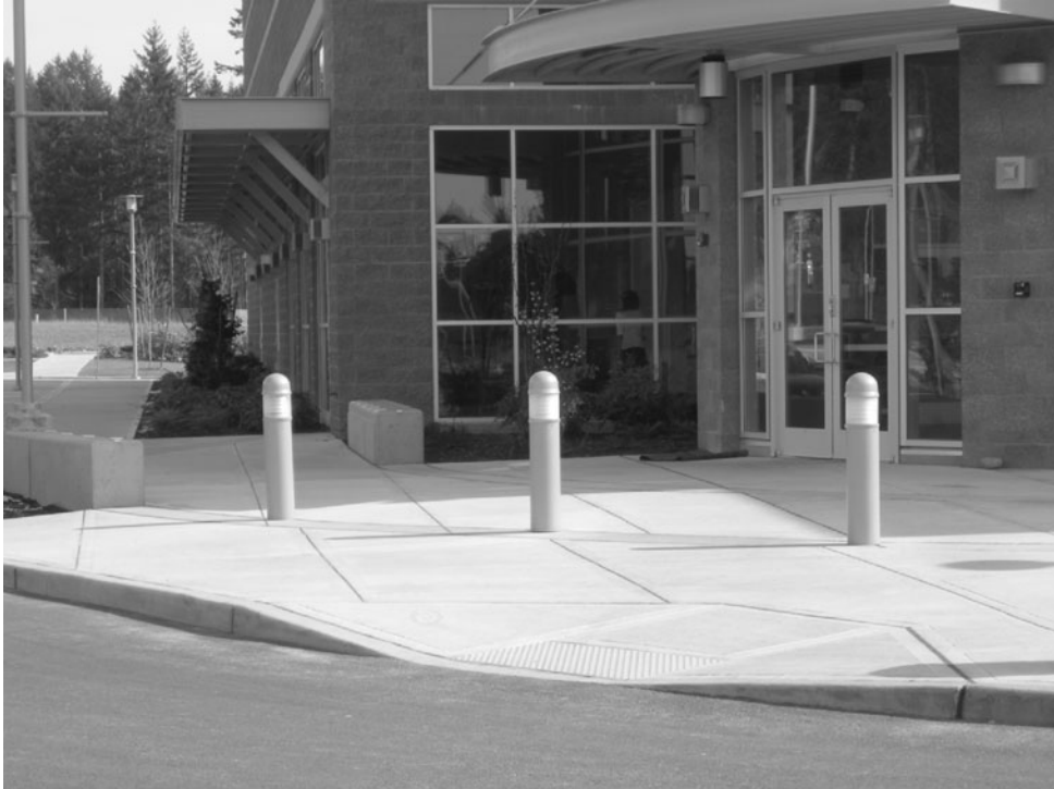
Figure 8-11 Bollards restrict vehicle traffic
