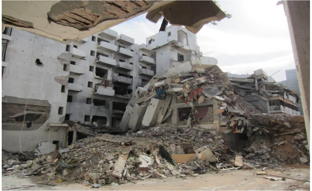
Apartment building struck on 16 September in Sirte © Amnesty International
