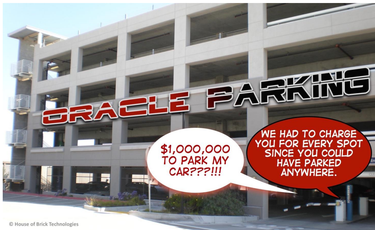
Figure 4: Oracle Parking Garage
