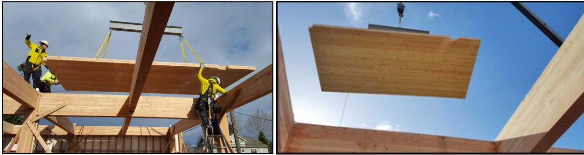
Figure 3 Installation of DR Johnson CLT panels at the Albina yard, Portland, Oregon (A). Photo credit, Kevin Cheung WWPA 2016. Installation of CLT Panels at Western Oregon University, Monmouth, OR (B), Photo credit Nicole Larsen.
