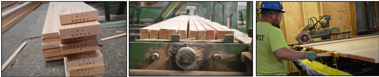
Figure 4 Lumber at the CLT facility is finger-jointed using MF resin and dried using radio frequency dryers.
