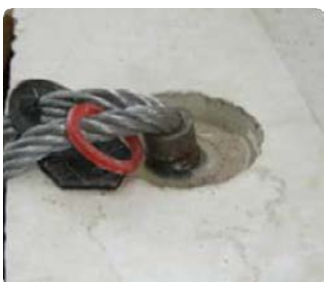
Wire slings bent over!
