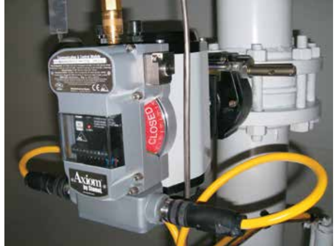
Axiom AMI with BPM module and electrical quick connectors.
